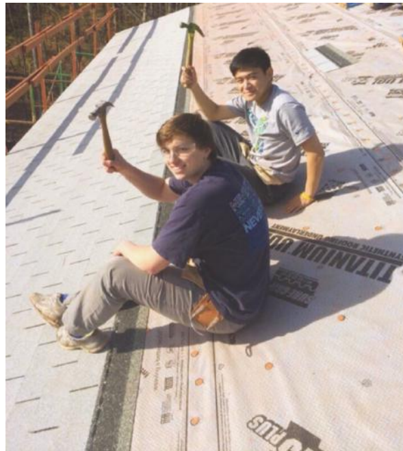
Brothers shingling the roof of a house for Habitat for Humanity
